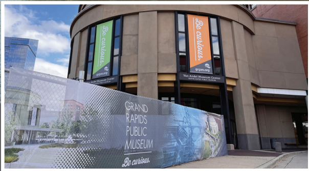
Rotunda with Construction Fencing
