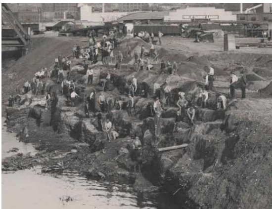
Floodwall reconstruction, circa 1905-1936 (178044.739) Flood walls and earth embankments were built to prevent more flooding. GRPM Collections
