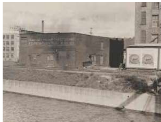
Floodwall reconstruction, circa 1905-1936 (178045.318) Flood walls and earth embankments were built to prevent more flooding. GRPM Collections
